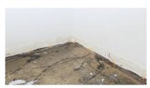
Installation should begin with a corner and proceed from the wall with the tongue facing away from the wall. Allow a minimum gap of 3/8" (10mm) for product expansion. Transition moldings or baseboards will cover the gap.
